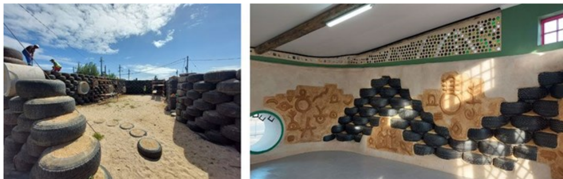
The new buildings will be constructed using sustainable building and circular economy principles, including rammed earth waste tyres from the Dunlop Ladysmith plant. Similar construction methods are pictured here at Cape Town's Delft ECD Centre built by Natural Building Collective.
