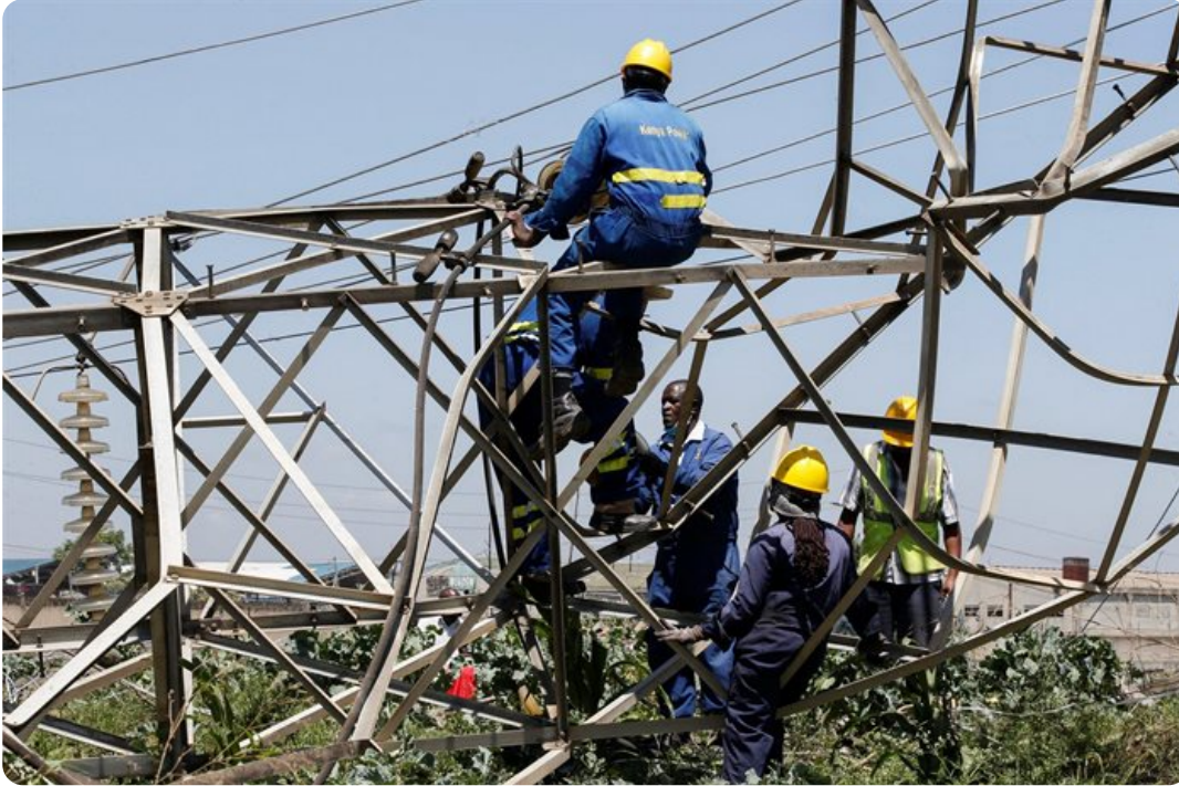
Technicians work on collapsed high voltage electricity transmission pylons from the Kambere hydroelectric dam in Embakasi district of Nairobi, Kenya, 12 January 2022. Reuters/Mnicah Mwangi
