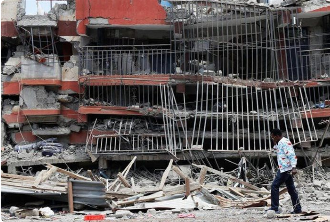
A man walks past the ruins of an apartment block that collapsed after 200 tenants were evacuated in Ruiru, on the outskirts of Nairobi, Kenya. Source: Reuters/Monica Mwangi
