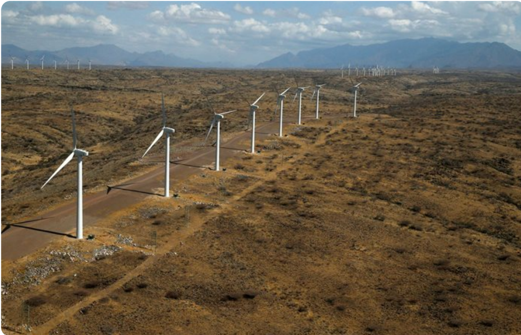
An aerial view of power-generating wind turbines at the Lake Turkana Wind Power project (LTWP) in Loiyangalani district, Marsabit County, northern Kenya. Source: Reuters/Thomas Mukoya
